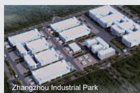
Zhangzhou Industrial Park
